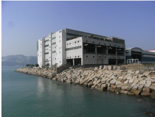
Photo 1 - The silt curtain was decommissioned off the seawall.
