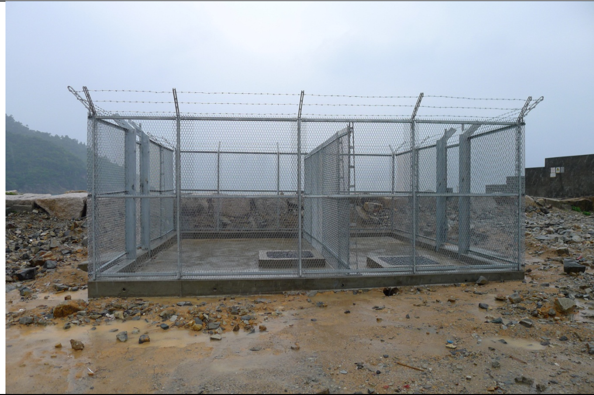
Photo 2 – BHM fence construction work completed
