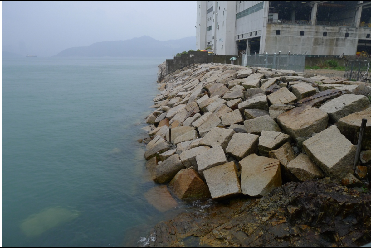
Photo 1 – No sediment plume observed in the sea adjacent to the Beach Manhole (BMH)
