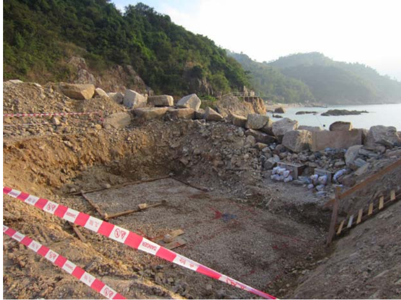
Photo 1 - Overall view of beach manhole construction site during site inspection.
